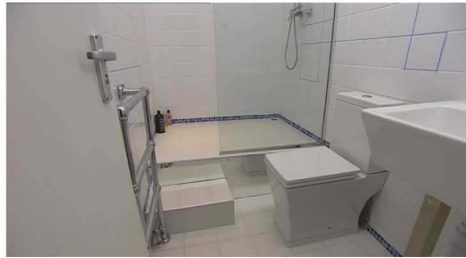
Bathroom after renovation
