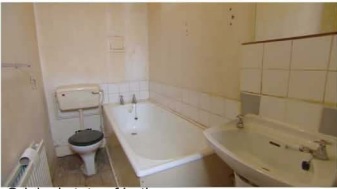
Original state of bathroom
